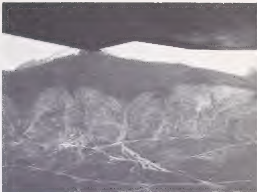
Figure 10.—Torrent flow deposit (center foreground) produced by failure of debris dam within the timber in center V-notch.
